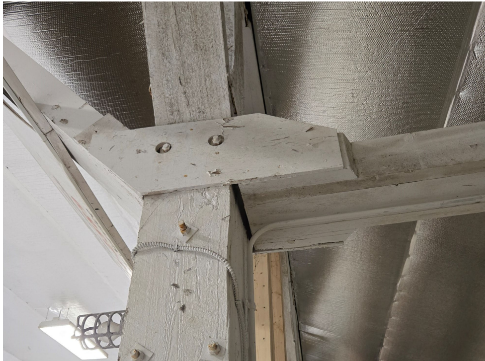
Photograph 5: Settlement effects at overhead structure
