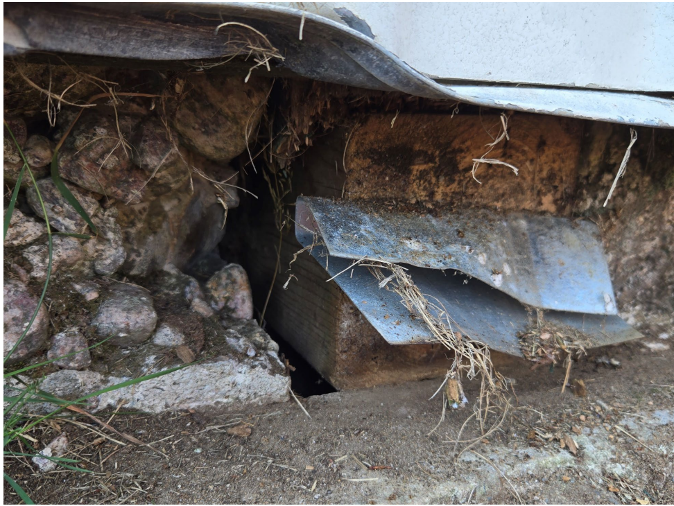
Photograph 7: Blocking at deteriorated column - exterior
