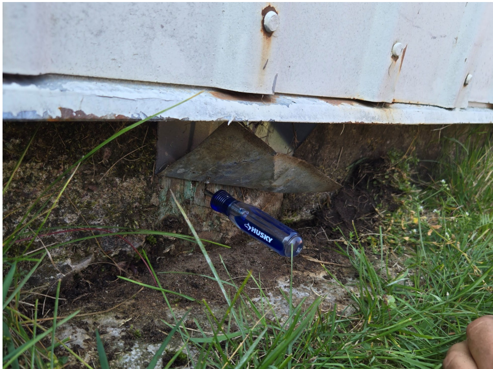
Photograph 6: Deterioration at original column - exterior
