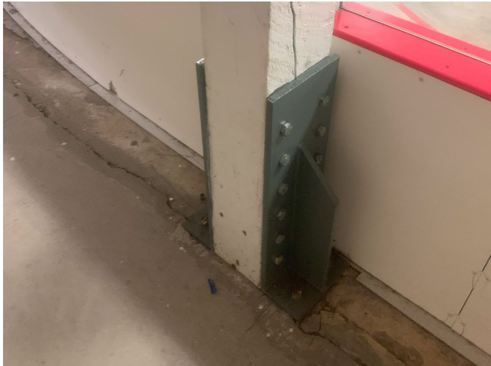
Photograph 3: Retrofit bolted steel plates - interior column
