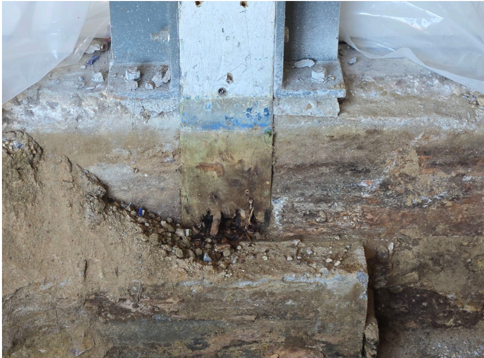
Photograph 1: Deterioration below slab - interior column
