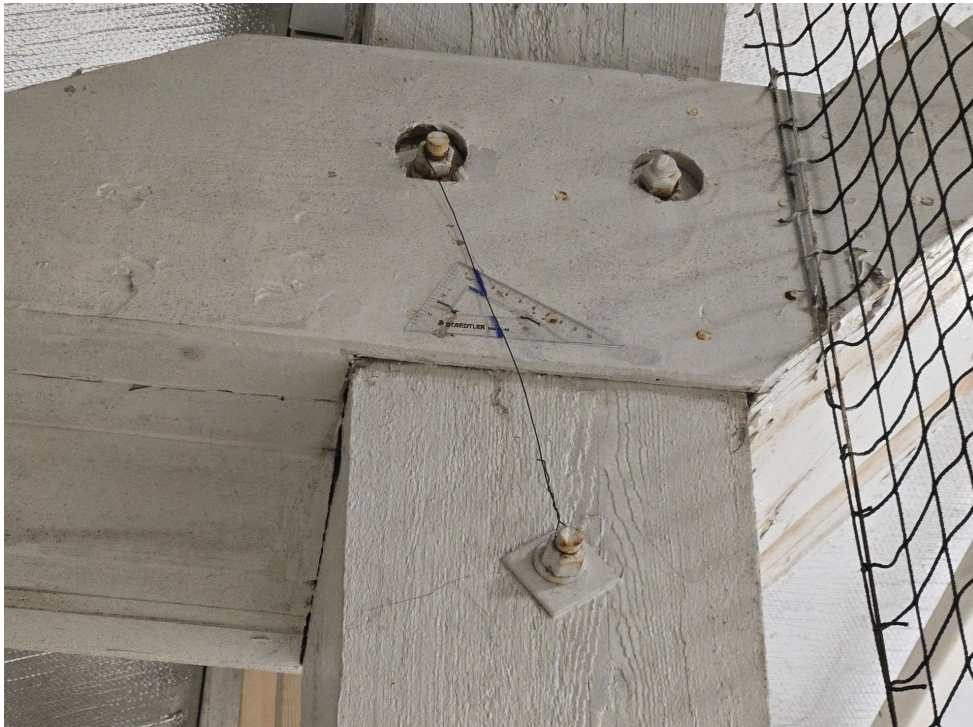
Photograph 9: Representative monitoring between column and adjacent structure
