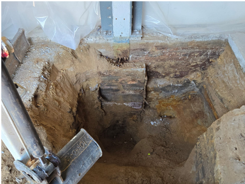
Photograph 2: Concrete pier adjacent foundation wall - interior
